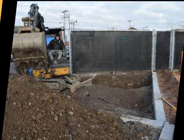
Step 2 PREPARATION level base, compacted
