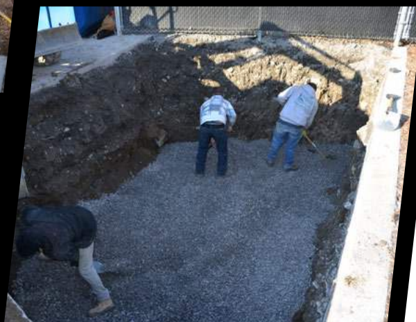
Step 2 PREPARATION level base, compacted
