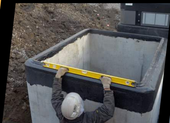
Step 3 INSTALLATION of the concrete insert
