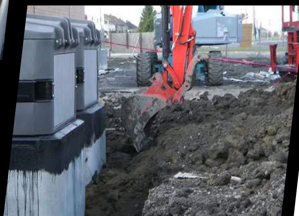
Step 4 REMBLAI crushed stone, gravel or sand
